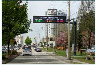
The City of Surrey announced its Advanced Traveller Information System (ATIS), dynamic messaging signs, to make traffic safer, improve flow, and reduce environmental impact. Three overhead, full color LED, Dynamic Messaging Signs are situated to provide alternate adjacent route choices for City Centre-bound drivers arriving from Highway 1 in the north and Highway 99 in the south. surrey.ca/TMC
